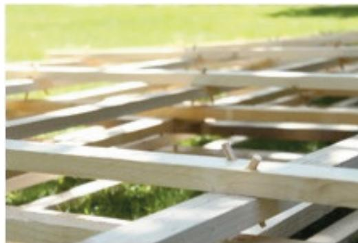
The wood pin – such a small object – became the very soul of the architectural concept of the team. Figure 2 shows the intersections of wood studs fasten by wood pins: pins are defined as “piece of solid material (as wood or metal) used especially for fastening things together or as a support by which one thing may be suspended from another” (Merriam-Webster, n.d.b, n.p.).
